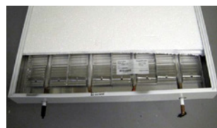
Fig. 3: Atrium H - Label location interior (under insulation, above water connection).
