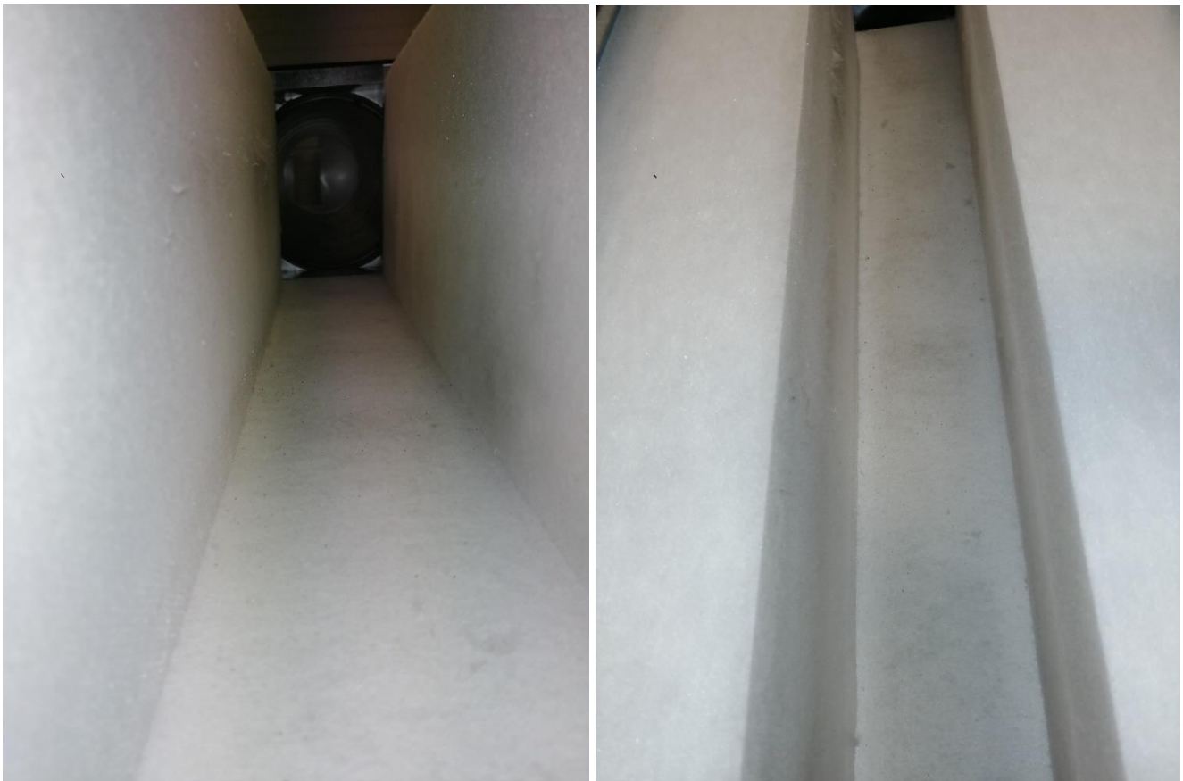
Figure 12. Straight duct: 1 brush cycle with steel brush: KVDPX-4 no1.
