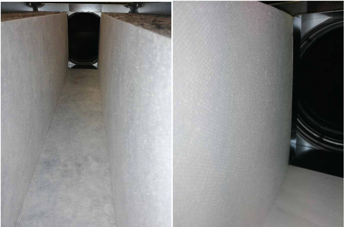
Figure 8. 90° elbow: 1 brush cycle: KVDPX-2 no2 and KVDPX-4 no2.
