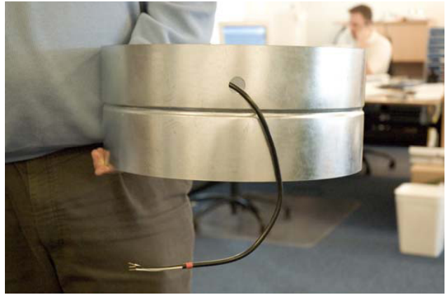
Put electric cable through drilled hole.
