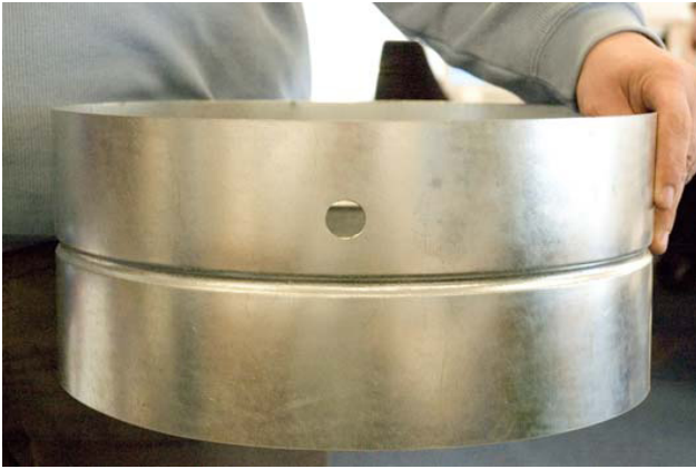
20 mm hole is drilled in duct where connection is wanted.
