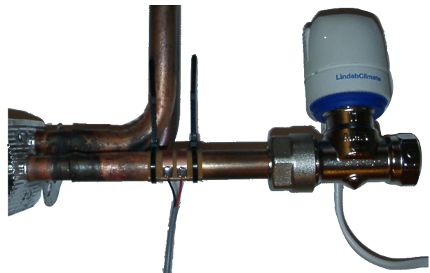
Figure 4 - Sensor fitted around horizontal smooth pipe and secured with 2 cable ties.
