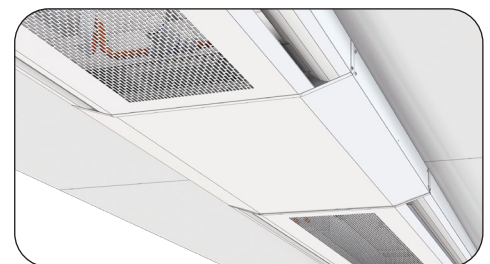
CC cover installed (screws inserted).
