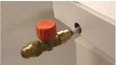
Notice! The connection pipes are internally soft-welded why it's not allowed to solder the panel to the pipes.
