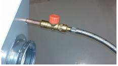
Notice! The connection pipes are internally soft-welded why it's not allowed to solder the panel to the pipes.
