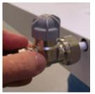
**Notice!** The connection pipes are internally soft-welded why it's not allowed to solder the panel to the pipes.
