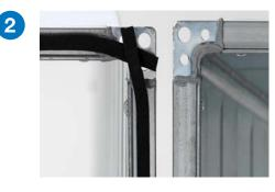
Apply the seal moulding (RJSM) to the inner edge of the connection profile. The seal moulding must cross over each other. The seal moulding is to be applied only to one of the two surfaces to be mated together
