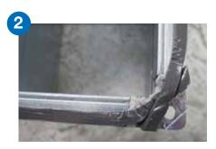
Apply the seal moulding (RJSM) to the outer edge of the connection profile. The seal moulding must cross over each other.
