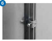
Assemble the Rectangular Joint Bolt Clamp RJBC over the flanges. To reach air tightness class B it is enough to have a distance of 700mm between the clamps. To reach air tightness class C a maximum distance of 400 mm is allowed.
