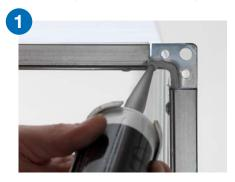
Mastic the countersunk part of the corner section (RJCL) and internally in the product's corners
