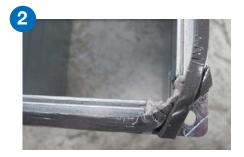
Apply the seal moulding (RJSM) to the outer edge of the connection profile. The seal moulding must cross over each other.
